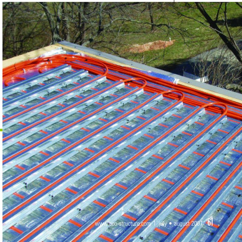
**THE CHESTERTOWN HOME MERGES THREE TECHNOLOGICALLY ADVANCED AND ENERGY-EFFICIENT ROOF SYSTEMS. IT FEATURES A SOLAR THERMAL WATER AND RADIANT-FLOOR HEATING SYSTEM, THIN-FILM PVs AND AN ENERGY STAR-RATED COOL METAL ROOF IN SLATE GRAY.**
